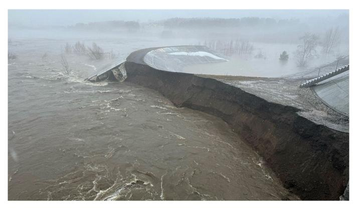
A partially collapsed protective dam in the city of Tomsk. tomsk.ru
