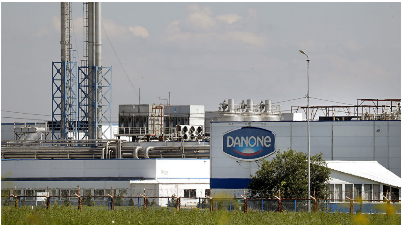
The Danone dairy plant in Chekhov, Russia. Maxim Shipenkov / EPA / TACC
