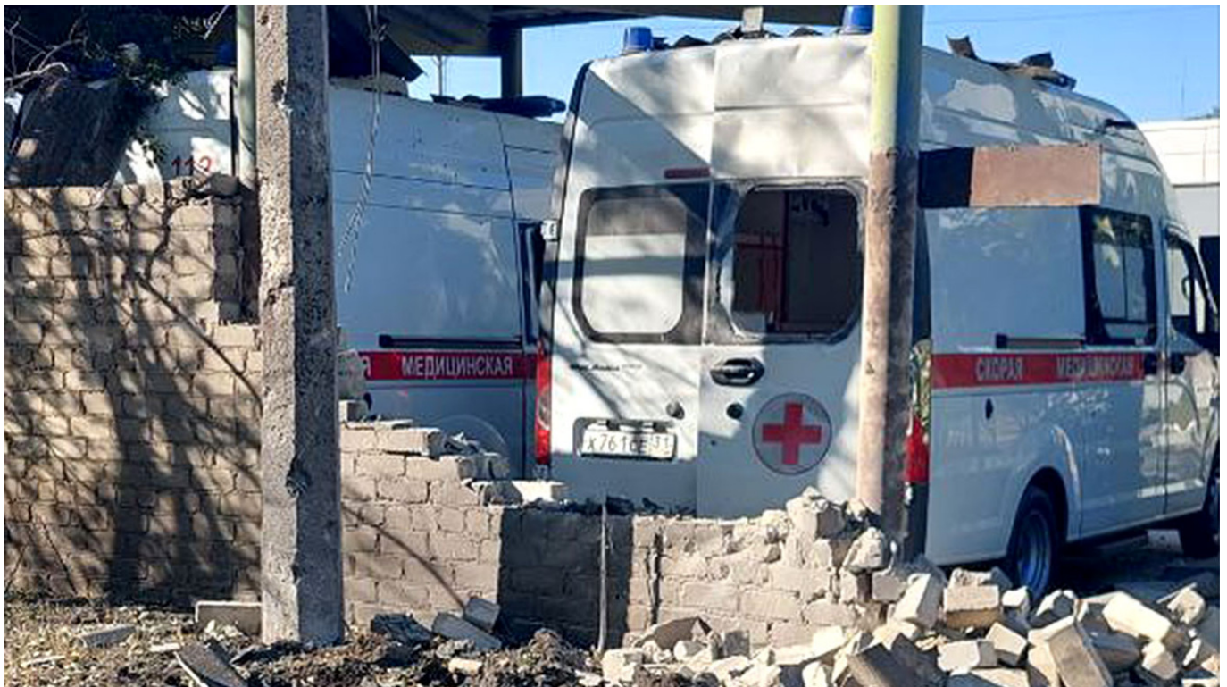
Shebekino Ambulance Substation Alexei Zhirov / VK
