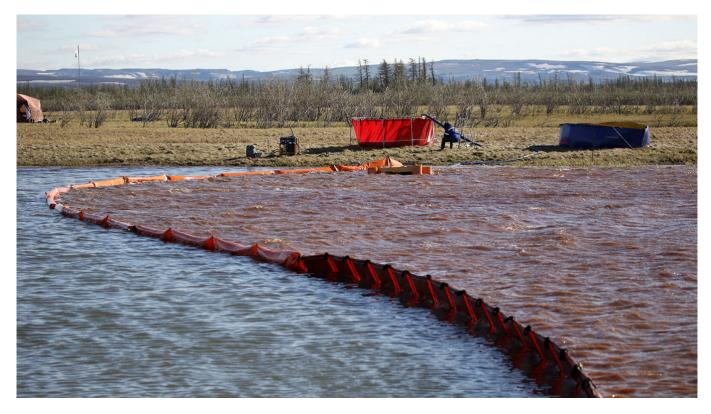
A containment boom deployed on a river during a major cleanup operation following the May 29 fuel spill at combined heat and power plant No 3, at least 20,000t of diesel fuel estimated to have spilled in total. **Kirill Kukhmar / TASS**
