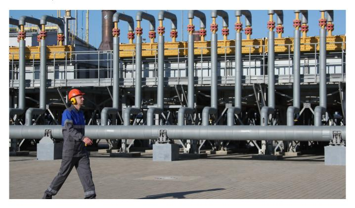
A worker walks by an air gas cooling unit at the Russkaya Compressor Station of the TurkStream gas pipeline in southern Russia's Krasnodar region. **Dmitry Feoktistov / TASS**
