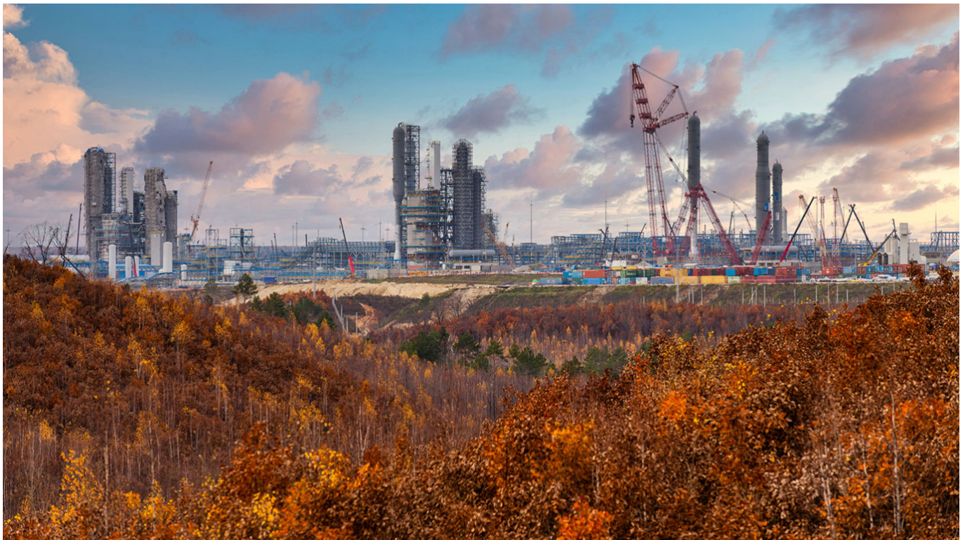
Amur Oil Refinery. Gazprom
