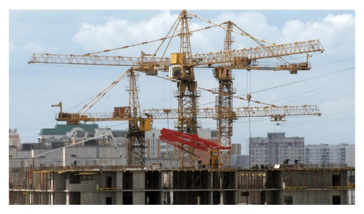
Many apartment blocks in Moscow are built quickly using prefabricated concrete panels that are simply set in place.
