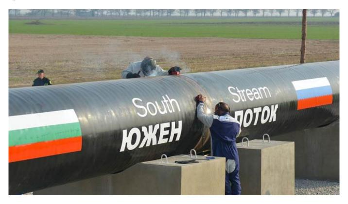
The first joints being welded at South Stream's Bulgarian section near the Rasovo CS site.
