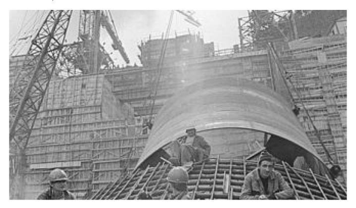
Workers at the Sayano-Shushenskaya power plant during the construction of a sluice pipe for a turbo generator unit.
