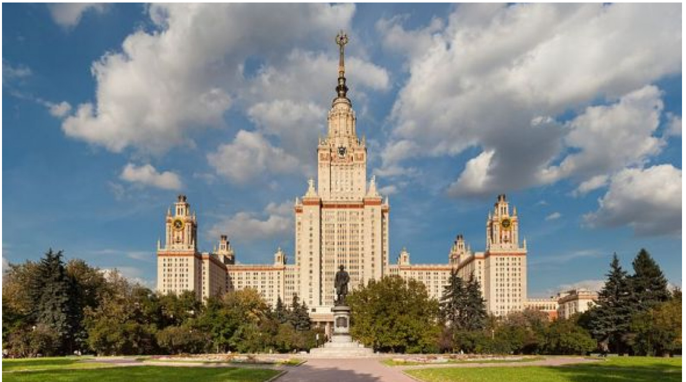
The main Building of MSU
