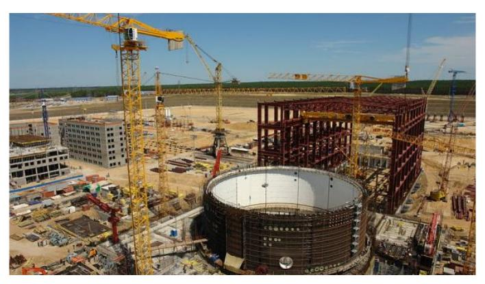
A 2010 photo showing the construction of unit one of the Novovoronezh Nuclear Power Plant II, scheduled for commercial operation in 2014. **Hullernuc**
