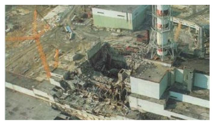
Taken shortly after the disaster, this Soviet government photo shows extensive damage to the main reactor hall, center, and turbine building, lower left.
