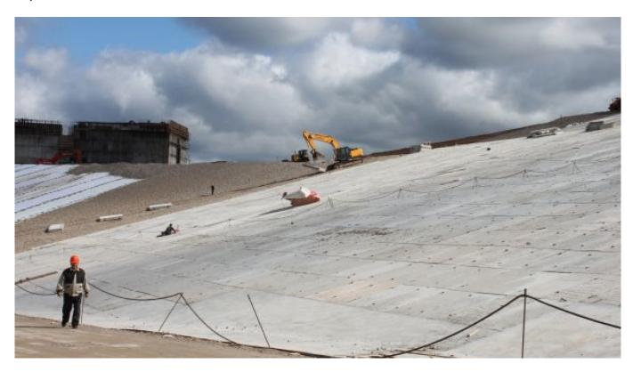
Workers building the plant's upper reservoir. The facility will generate electricity via the downward flow of water. **Anna Butusova**
