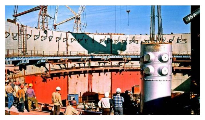
Part of a VVER 1000 nuclear reactor — the model Rosatom is expected to market to Hungary for its Paks power plant — being installed at the Balakovo nuclear power plant in the Saratov region.
