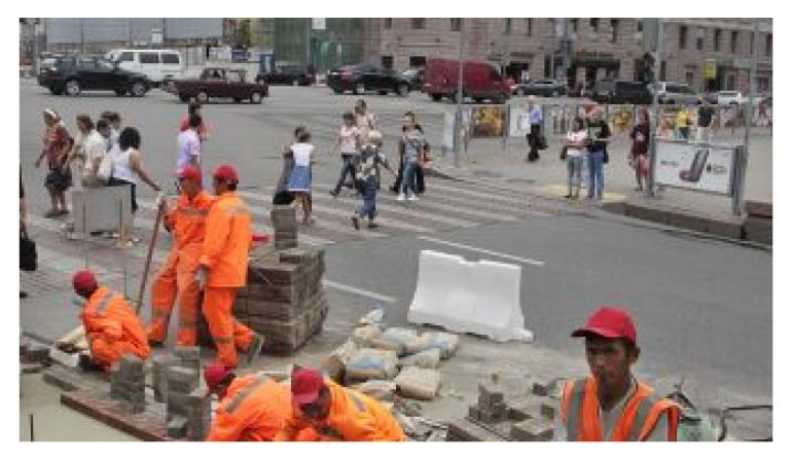
Tajik workers replacing an asphalt sidewalk with bricks near Pushkin Square. Brick makers have run out of bricks. **Igor Tabakov**
