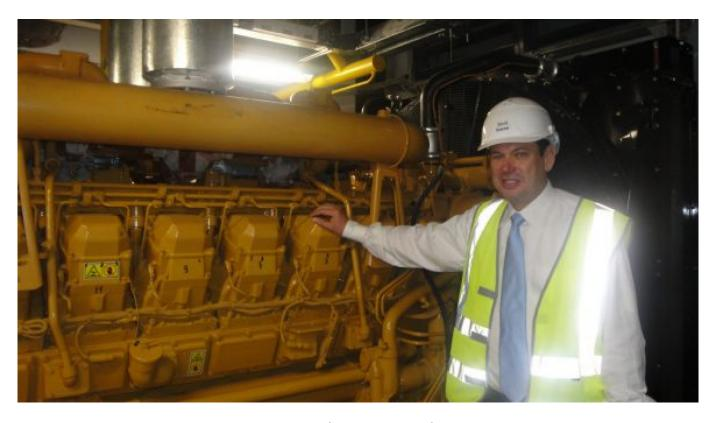
DataSpace's six generators can keep it running for three days of power outage, in line with Tier III certification. **Lena Smirnova**
